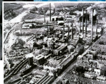
The site of RWE's first power plant will soon be home to the new Midstream building
