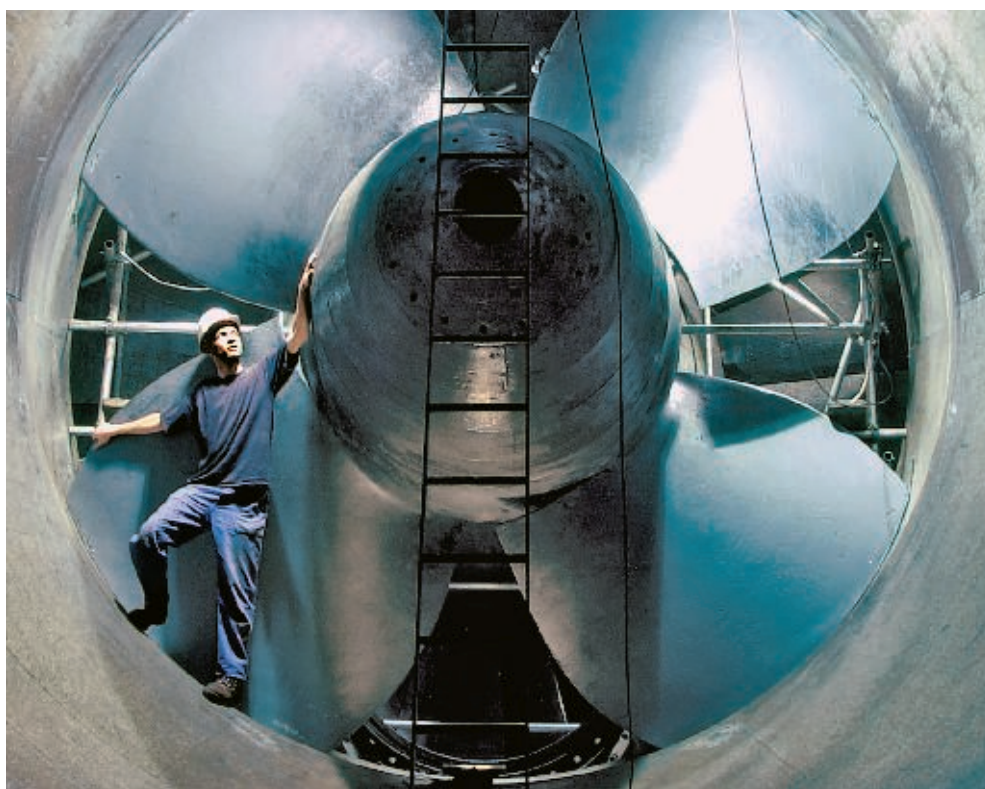
The Radag run-of-river-power plant will be upgraded by a Kaplan turbine
