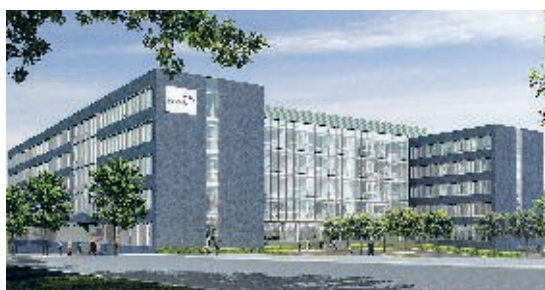
The new office building at Altenessener Straße
